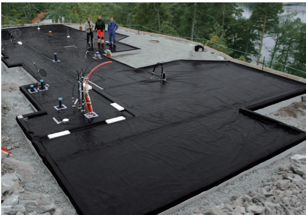
DELTA®-RADONSPERRE the barrier against radioactive radon entering from the ground.
